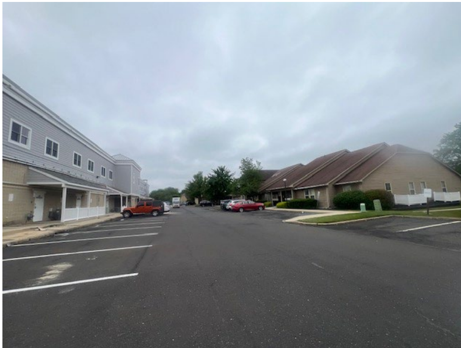
Photo 6: Representative view of the eastern portion of the site.
