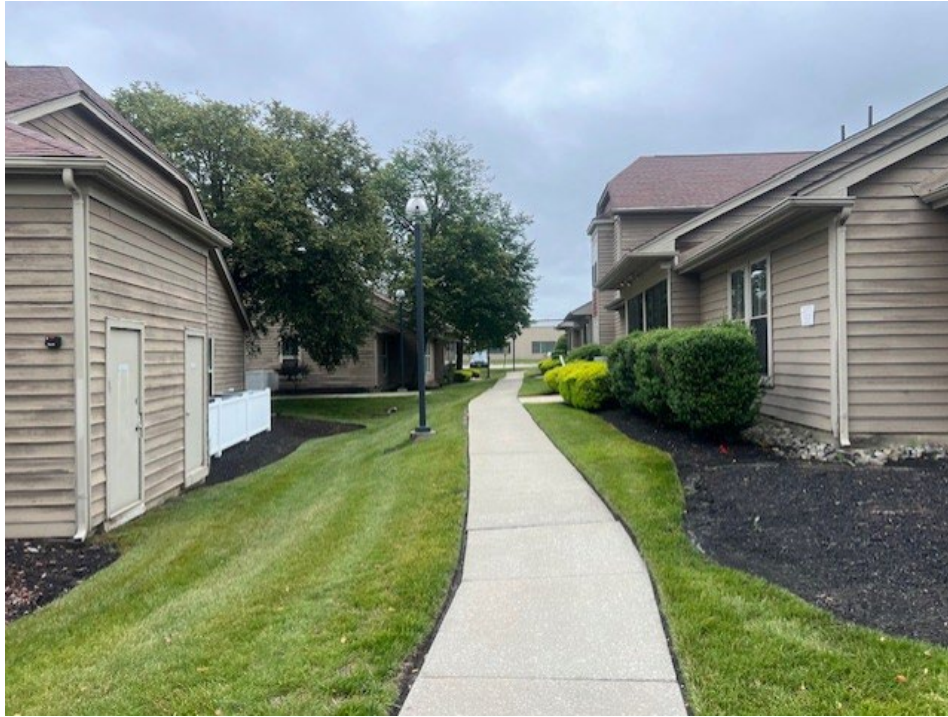
Photo 7: Representative view of the central portion of the site.
