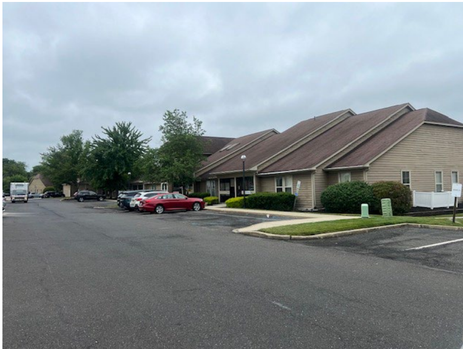
Photo 4: Representative view of the central portion of the site.
