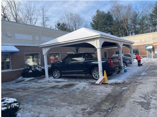
PHOTO #3 NORTH ELEVATION
