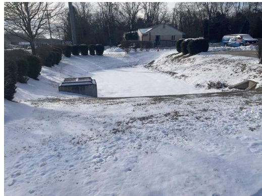
PHOTO #24 STORMWATER DETENTION BASIN
