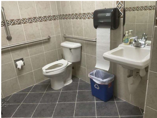
PHOTO #9 CUSTOMER RESTROOM
