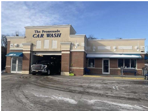
PHOTO #5 EAST ELEVATION
