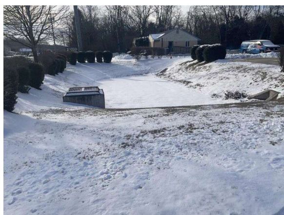
STORMWATER DETENTION BASIN
