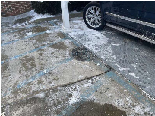
PHOTO #21 RECLAMATION TANK (1 OF 4)
