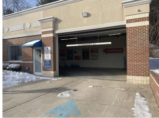
PHOTO #2 NORTHWEST ELEVATION
