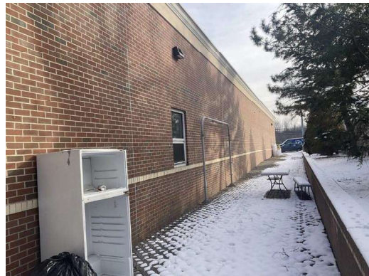
PHOTO #6 SOUTH ELEVATION
