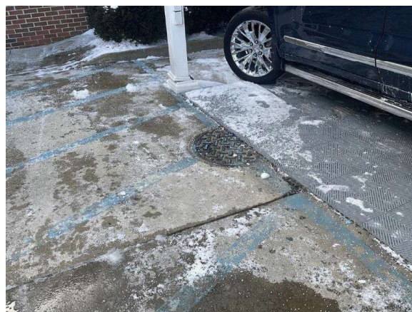
RECLAMATION TANK (1 OF 4)
