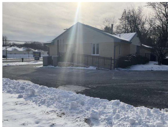
ADJOINING SOUTH COUNTY LINE VETERINARY HOSPITAL
